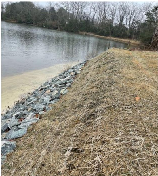
Rip rap complete. Top planted with native river oats (January 2021)
