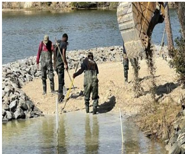
Figure 2: Building up sand nourishment on the West Sill
