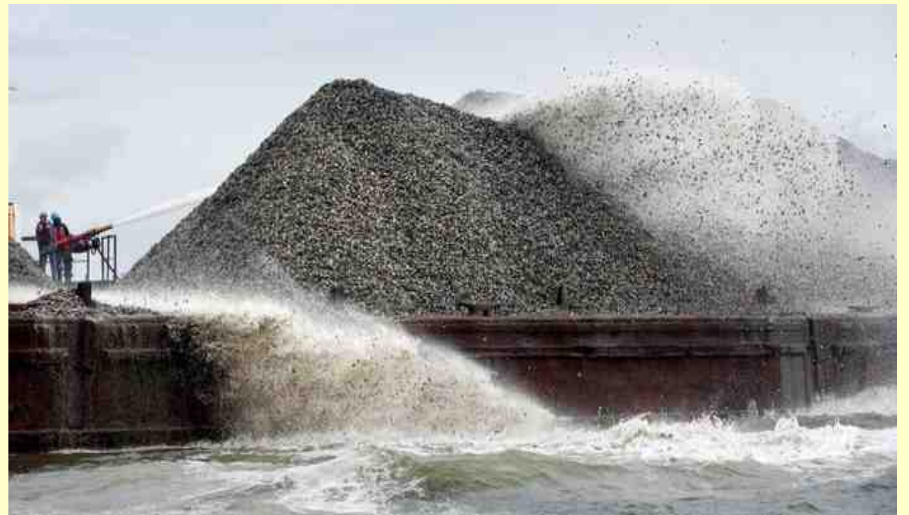
Water cannons spray fossilized shell on working oyster grounds on the James River.
