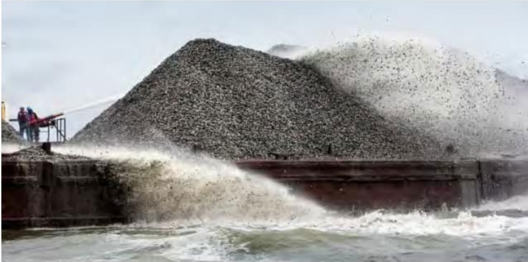
Water cannons used to spray fossilized shell on working oyster grounds on the James River.
