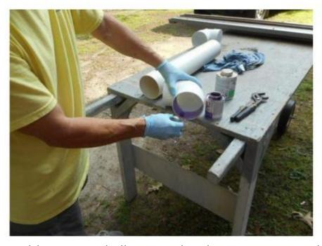
After adding second elbow on the short pipes, press hard on a table to align the elbows so the long pipes will be parallel.
