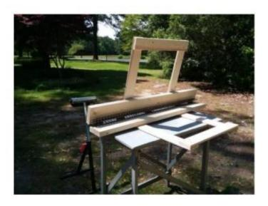
First a ~3/8 in. chamfer is cut along each 2x6. This is to make room later for the hinge barrels.
