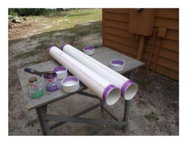
Prime the pipe ends and cap walls with purple primer. Then Coat the pipe ends and cap walls with heavy-duty PVC cement. Push the caps all the way on the pipe with a ¼ turn. When placing the cap on the opposite end, hold down for 15 seconds so the air pressure will not push the cap out.
