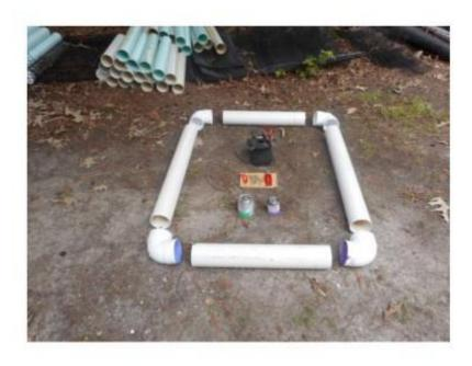
Apply primer to elbows and pipe. Add heavy-duty cement one corner at a time. Work fast while the cement is wet.
