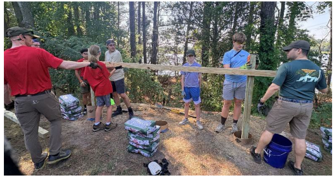
Matt Paluskiewicz, Mike Paluskiewicz, Nikolai Szymanski, and Jamie Johnson aligning the right post to the left post before concrete is poured, with (starting from left again) David Jimenez, Andrew Poler, Issac Valdez, and Davis Graham standing by.
